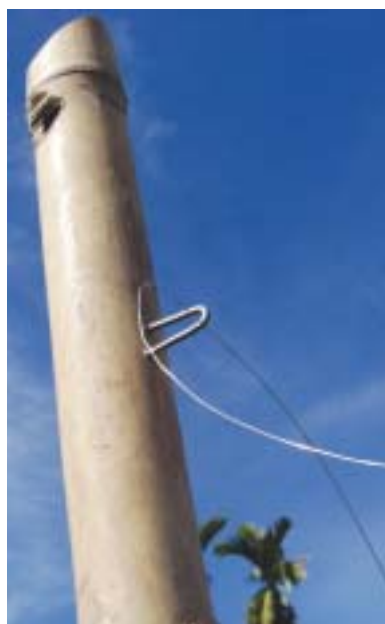
Pass the GI wire through the eye of the hook
