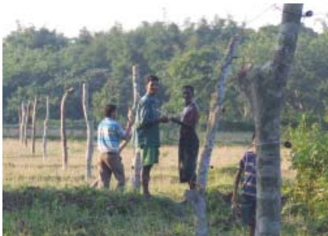
Place intermediate posts 10 metre apart and make every 11th post a strain post on long straight stretches
