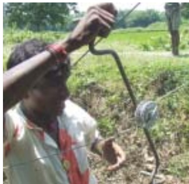
Tighten the wires by winding it on wire strainer
