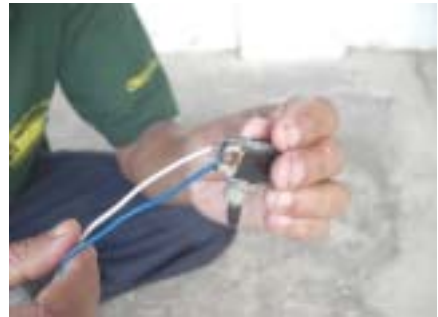
Attach wire to the switch
