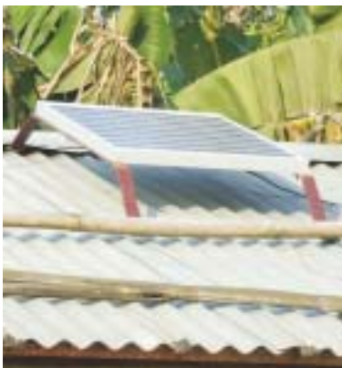
Solar panel on the roof
