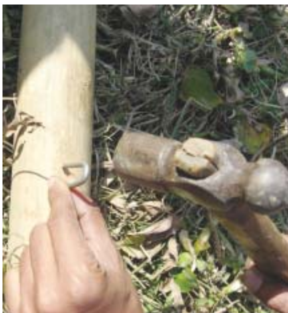
Drive the U-nail into the pole at 2.1 m height
