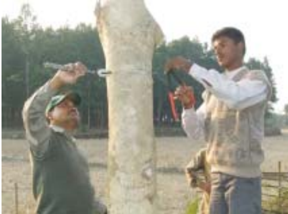
Fix strain insulators and tension spring on strain and corner posts; here a tree is being used as a strain post
