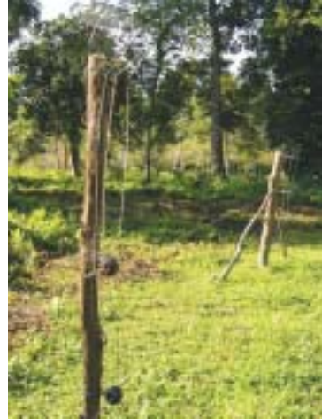
Fix reel insulators on intermediate posts
