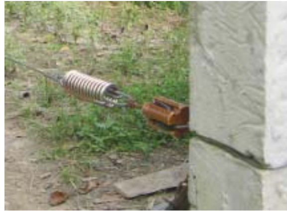
Make the strain insulator ties strong; use insulation sleeves and fix the spring only on one end of each wire length
