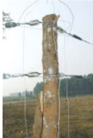
Jumpers and vertical post protection wires on strain post (2-strand fence)
