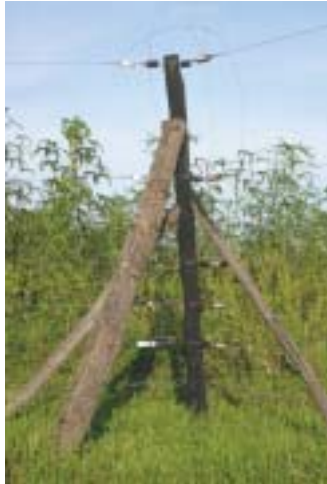
Corner post: notice the supports
