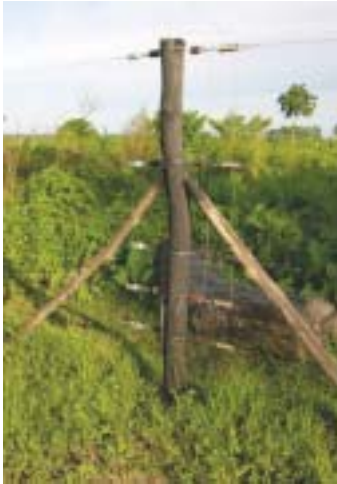
Strain post (5-strand fence)
