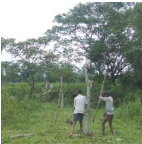
Fix posts approx. 0.75 m into the ground
