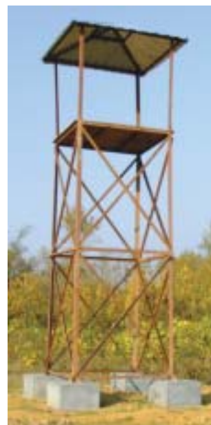
Steel watch tower with GI sheet roof
