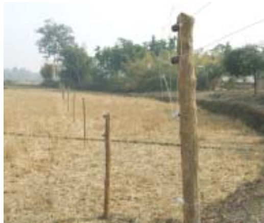
2-line power HEC fence in AHP project area
